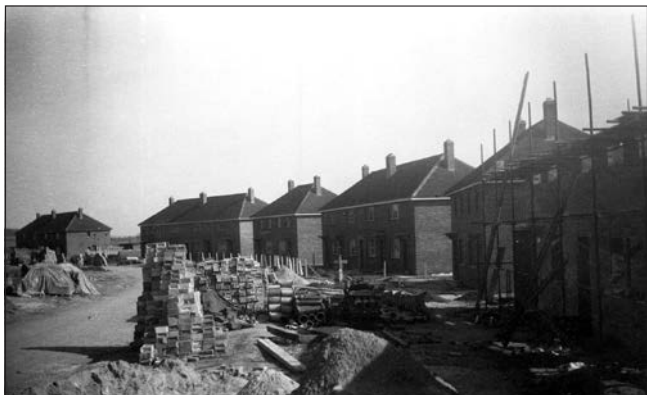
Construction of homes in Foster Road, c. 1946. Cambridgeshire Collection (stop 14).
